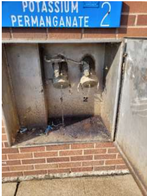
Existing Pot Perm Truck Unloading connections that continue to get used.
