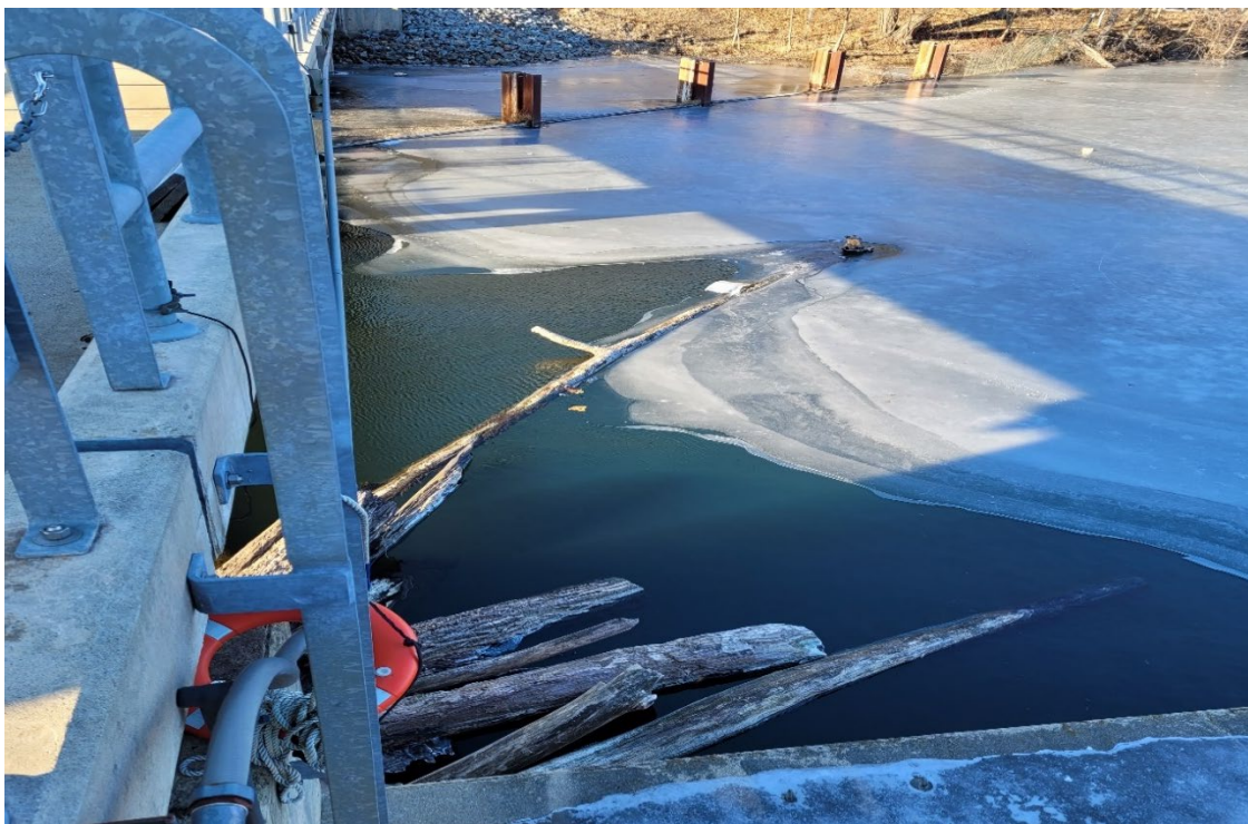
Photo #3: Upstream side of Tainter gates (looking north). Note: Large debris obstructing the path to the gate.
