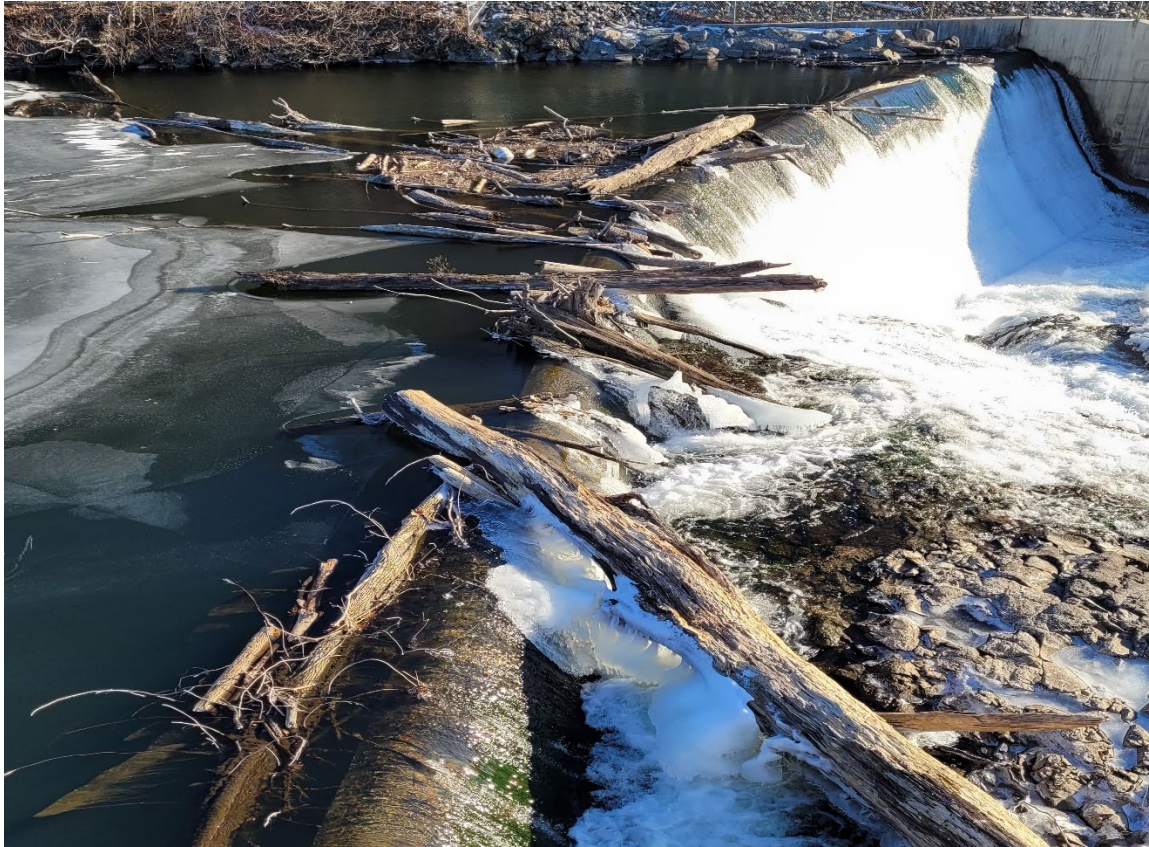
Photo #3: Southern spillway. Note: Large amounts of downed trees obstructing spillway.
