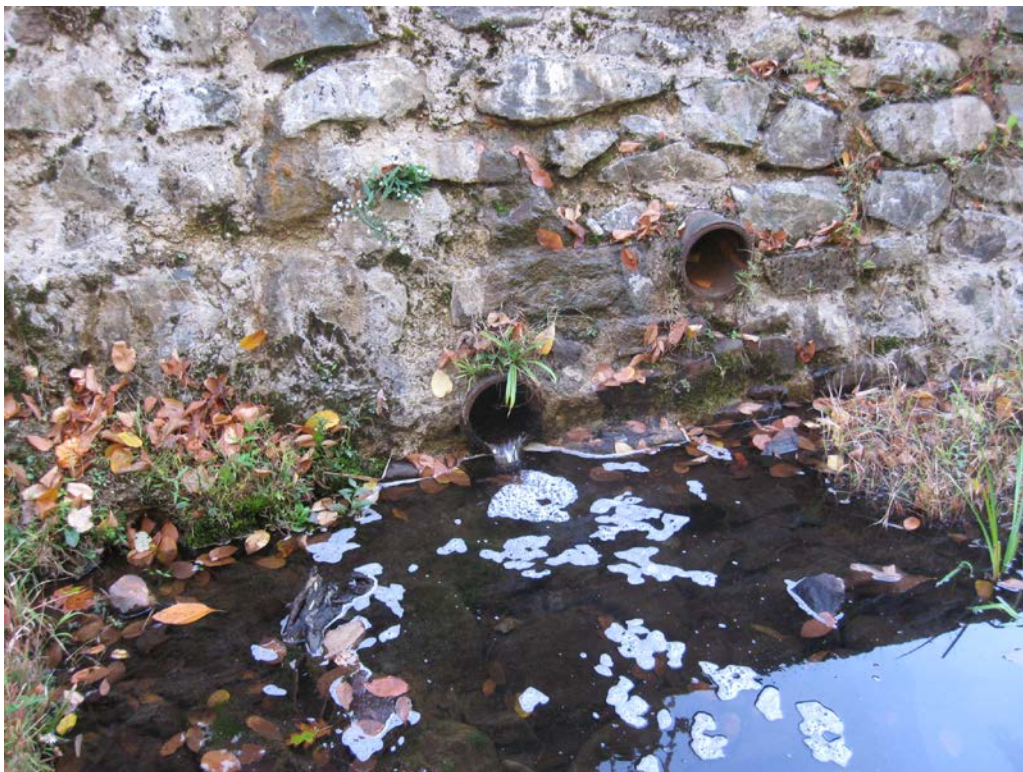
Photo 15: Low-level outlet discharge pipes at the downstream face of the dam.
