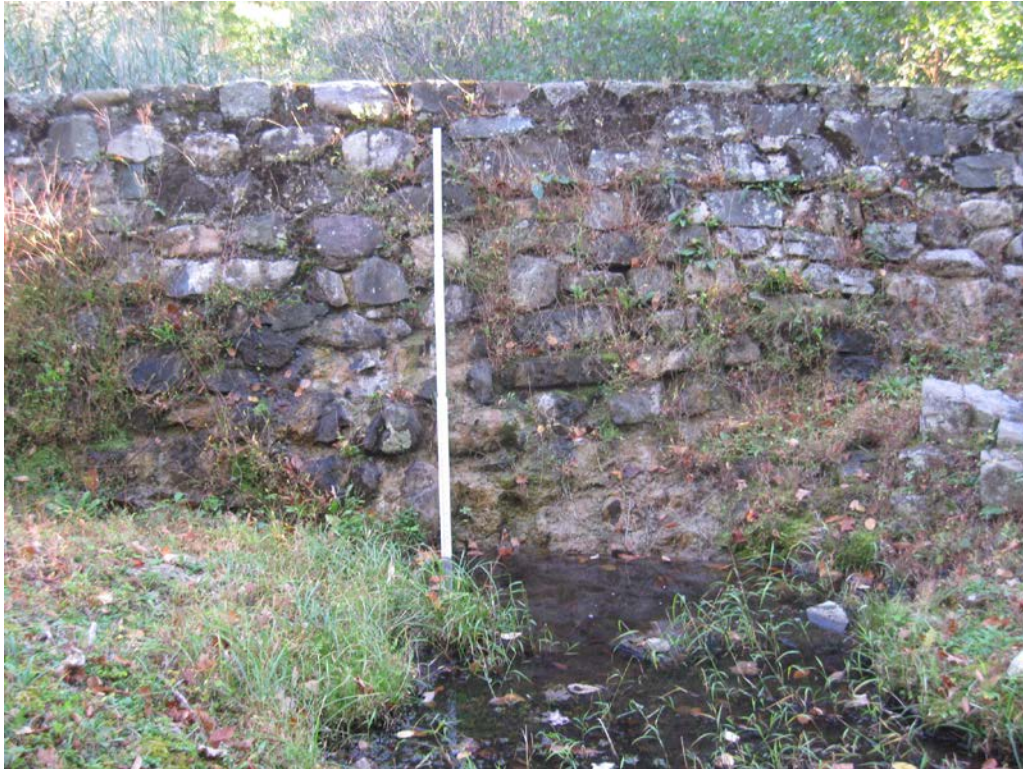
Photo 5: Downstream face of the dam near the left abutment. Note the swale at the downstream toe.
