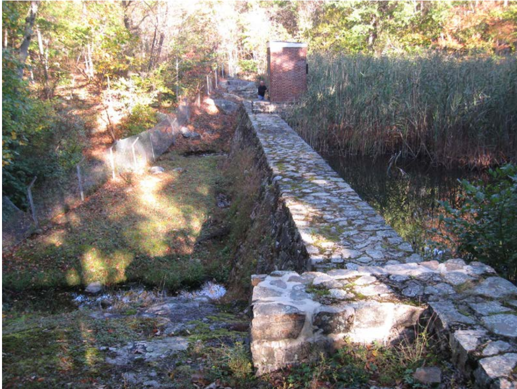
Photo 1: Overview of the rubble masonry dam from the left abutment. Note the heavy stand of phragmites upstream of the dam.
