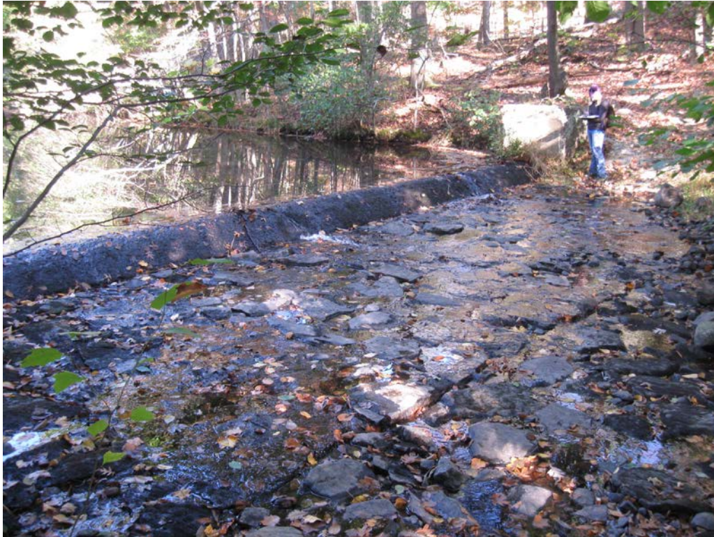
Photo 13: Overview of spillway over flow weir, left abutment and downstream apron.
