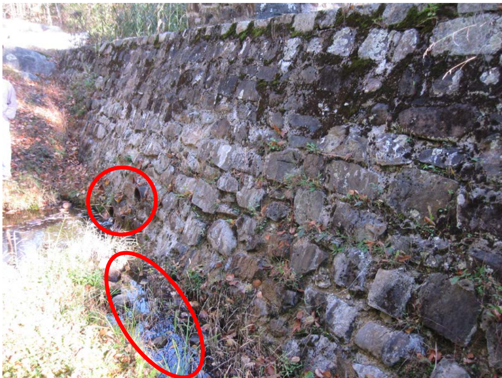
Photo 4: View of downstream face of the dam near looking towards the right abutment. Note standing water in the scour hole at the downstream toe of the dam. Also note the location of the low-level outlet discharge pipes.
