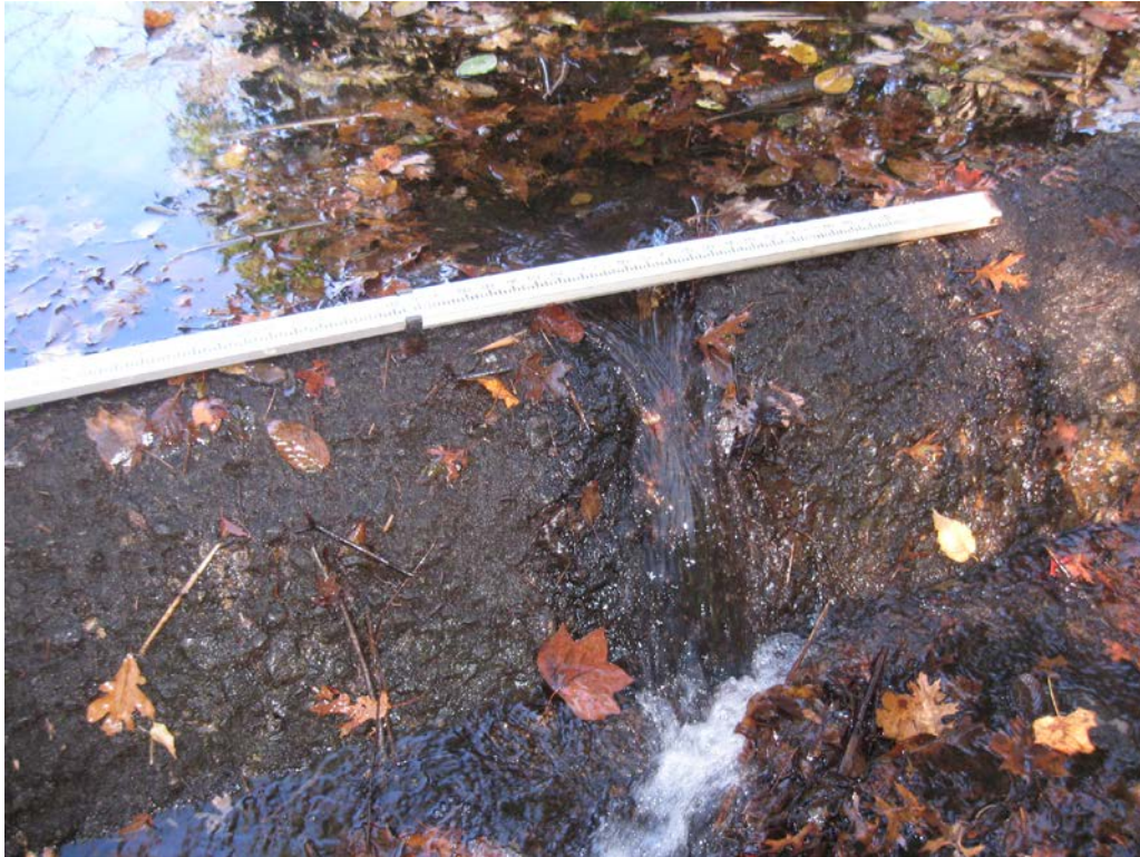
Photo 11: Closeup of the larger of the two cracks in the overflow weir crest.
