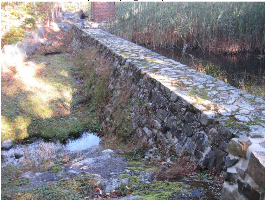
Photo 2: View across the crest and downstream face of the dam from left abutment. Note the vegetation growth on the downstream face.
