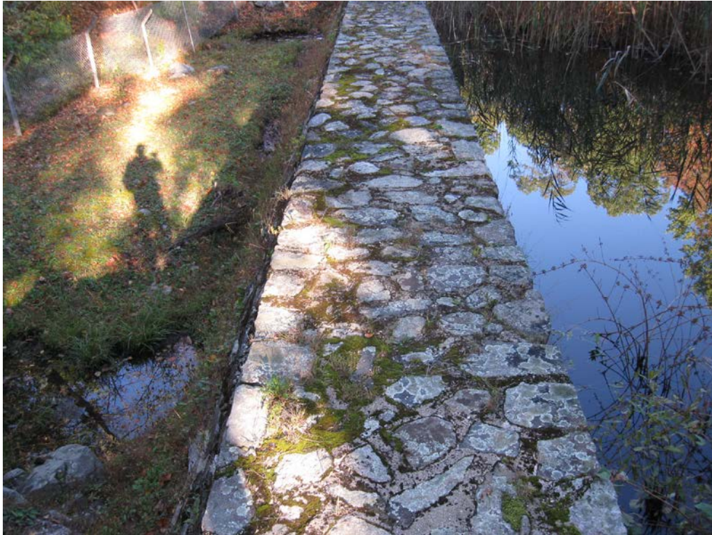
Photo 7: View of the dam crest looking right. Note the intact condition of the stone masonry.
