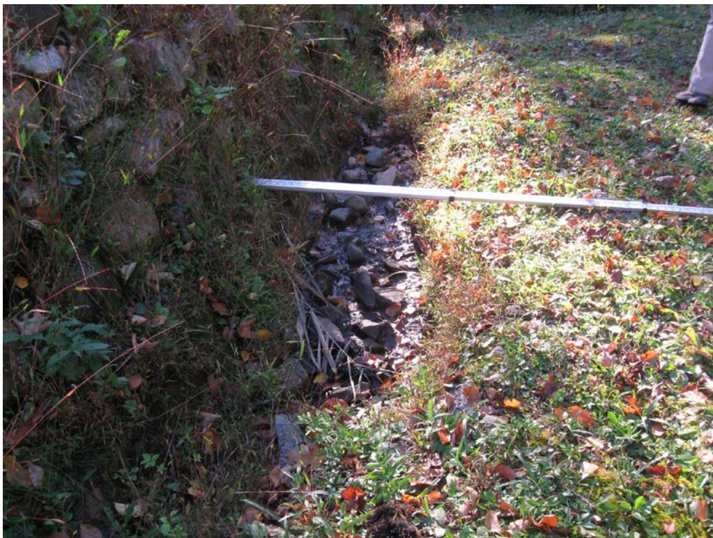
Photo 6: Closeup of scour hole, near the center of the dam, with standing water at the downstream toe.
