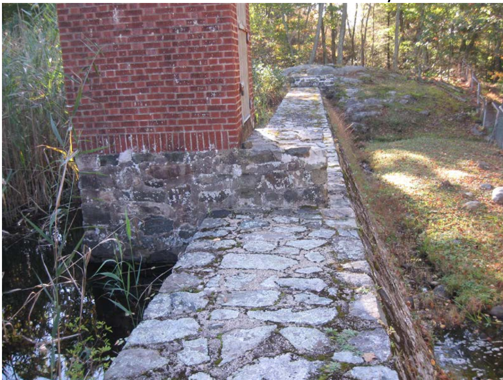
Photo 8: View of crest of the dam and gatehouse for the low-level outlet valves.
