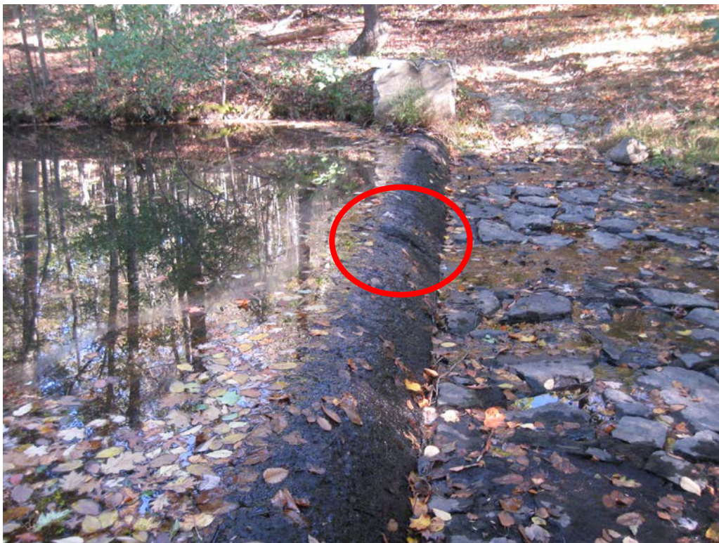
Photo 10: Looking left across the spillway entrance channel and spillway overflow weir crest. Note the crack in the spillway.
