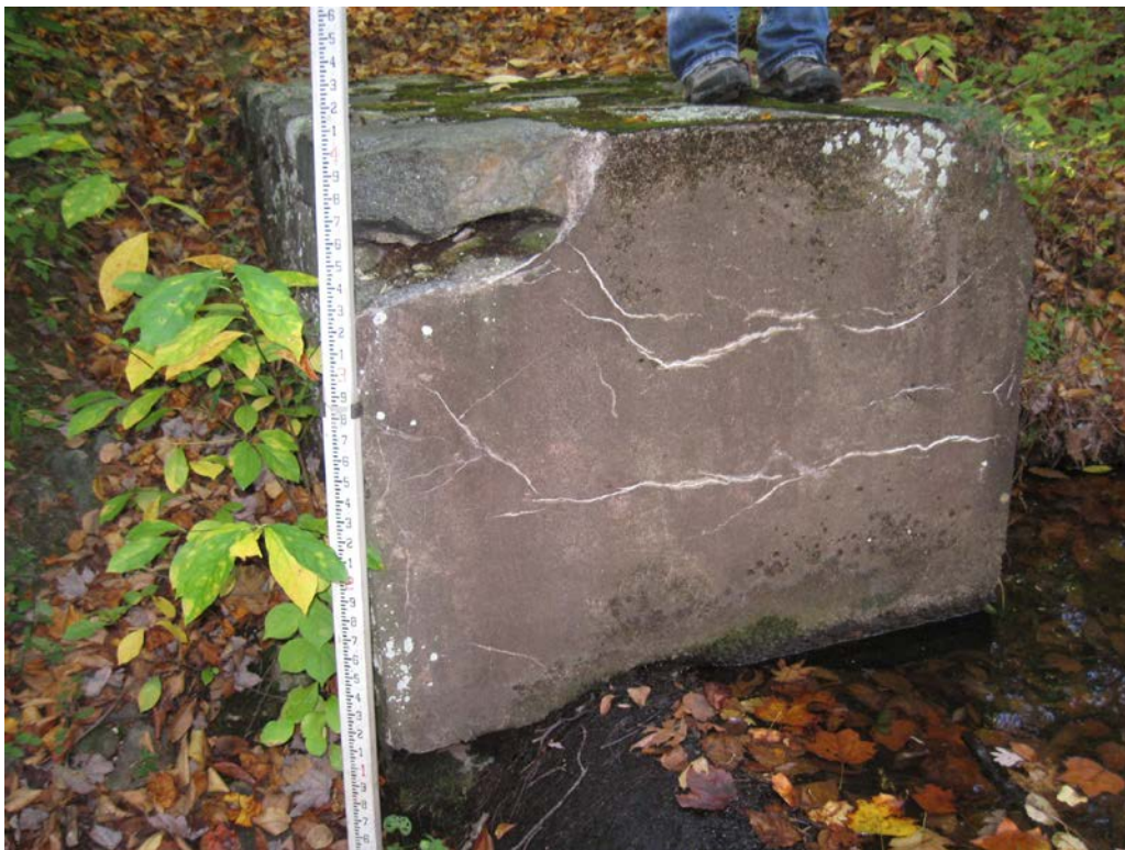
Photo 12: Right spillway overflow wier training wall. Note the missing mortar at the top of the wall.
