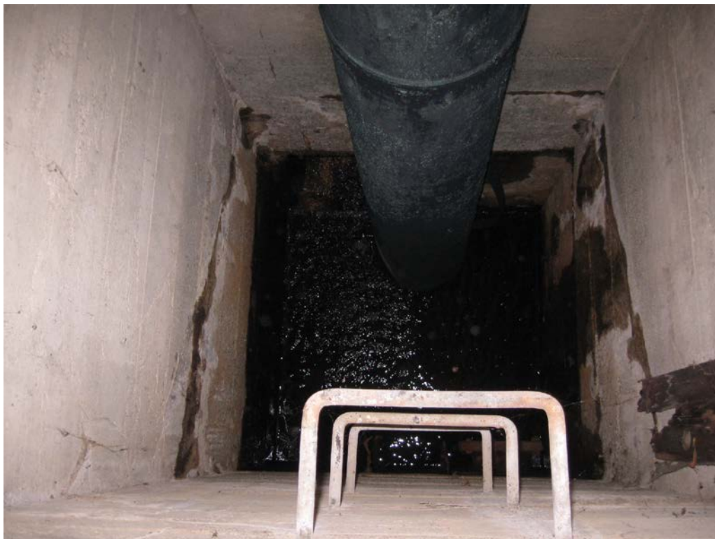
Photo 17: Interior of gatehouse. Note the copper cylinder gaging well.
