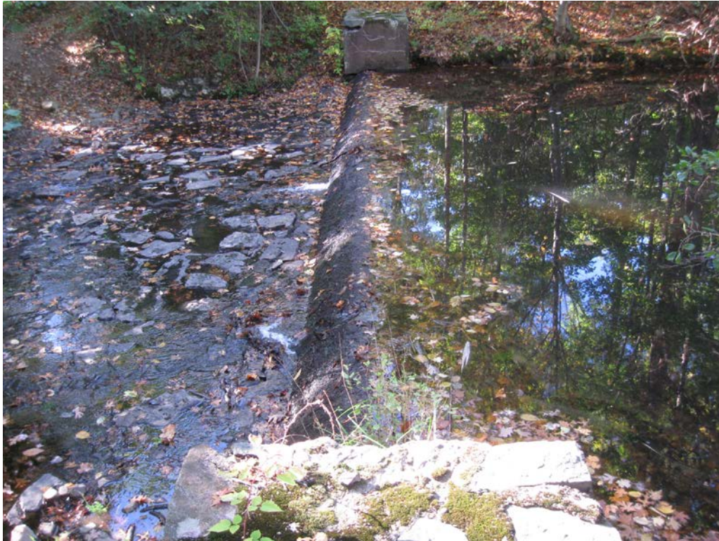
Photo 9: View across the spillway entrance channel and spillway overflow weir crest.
