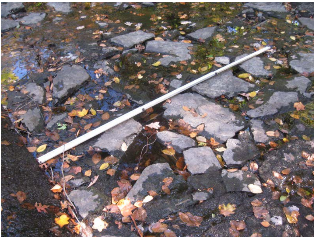
Photo 14: Closeup of stone masonry apron.
